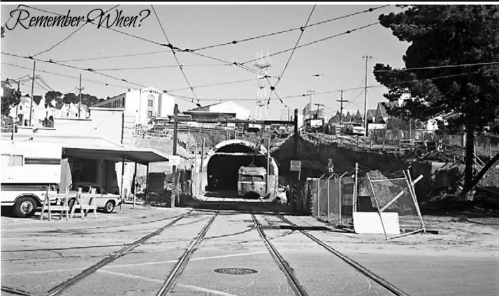
Reconstruction of West Portal Station to Expand Passenger Waiting Area and Raise Platforms for New Muni Metro System and New Light Rail Vehicles in 1976 and 1977. November 16, 1976 Reproduction by permission of SFMTA Photo Gallery
